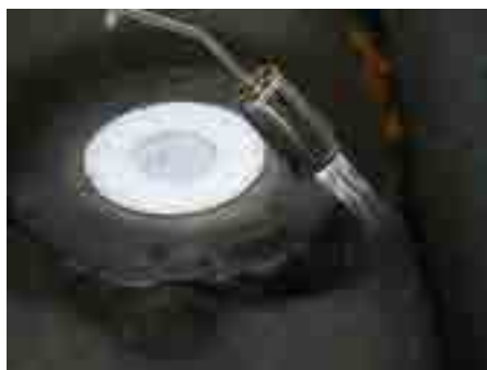
2. Weld the prefabricated bitumene flange with the local bitumene waterproofing
