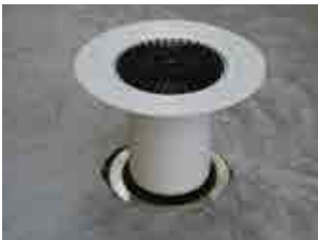
7. Put the extension HL350.0 on the gravel guard HL160
