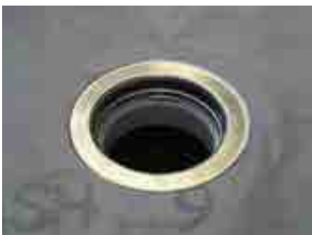
10. Clamp the fleece on the flange with the stainless steel ring
