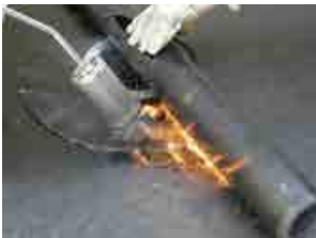
4. Connect second bitumen layer with the bitumen flange of the drain
