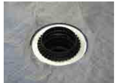
6. Remove lid cover, apply the fleece, insert gravel guard HL160
