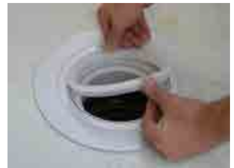
9. Insert the transparent plastic ring in the groove of the flange
