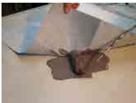
7. Apply the liquid waterproofing
